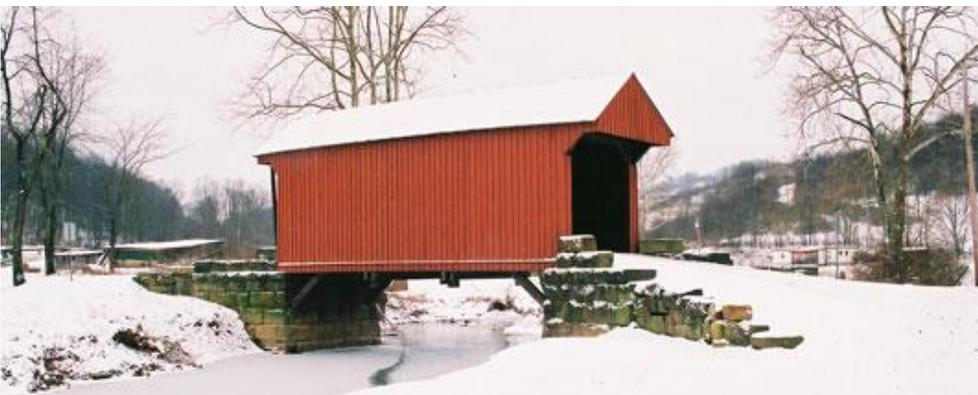
Built by John Sprigg for \$567 in 1903, this 12-foot-wide, 39.25-foot-long queenpost truss bridge carries vehicles on Lewis County 19/17 over Right Fork of West Fork River.
