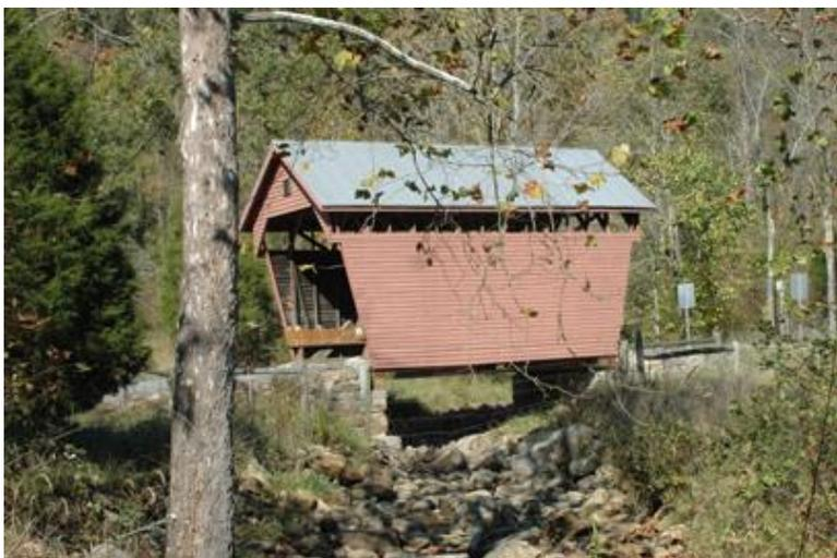
West Virginia's smallest covered bridge is just over 13 feet wide and just under 24.5 feet long and still carrying traffic. Built by Robert Arnott in 1912 at a cost of \$365, the queenpost truss carries Monroe County 219/11 near Lillydale. The bridge was renovated in 2000 by Hoke Brothers, Inc. of Union, WV for \$248,692.
