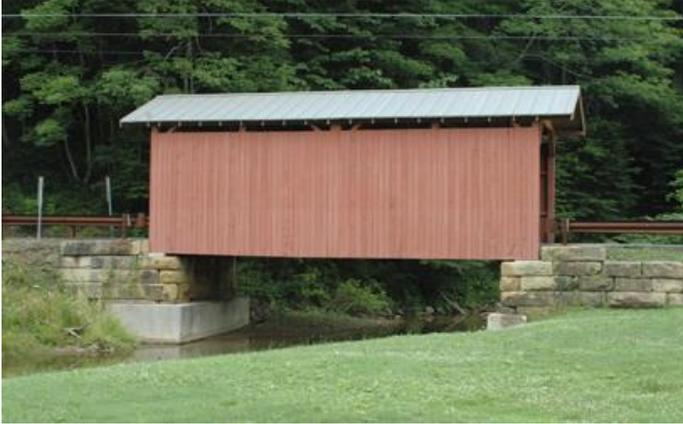
Located on Wetzel County 13 near Hundred, this kingpost truss is 12.75 feet wide and 36 feet long and still carrying traffic. Few details of its 1880 or 1881 construction are known. Lone Pine Construction, Inc. of Bentleyville, PA completed renovation of the bridge in 2001 for \$218,409.
