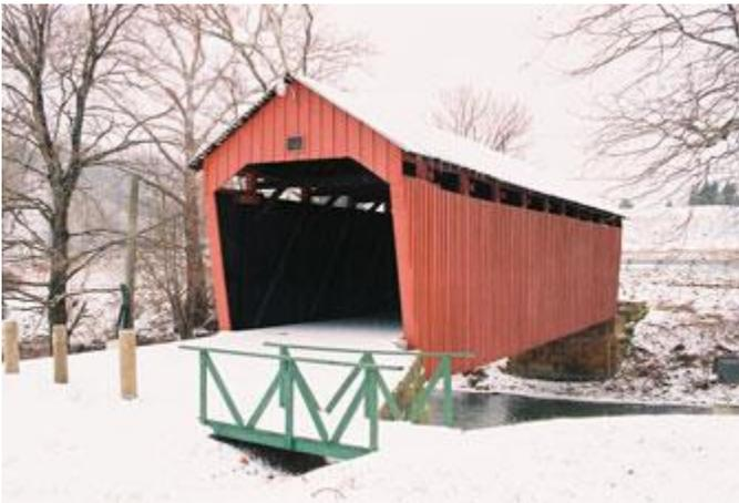
A 14.25-foot-wide, 75-foot-long multiple-kingpost truss, this covered bridge built for \$1483 by Asa Hugill in 1881 once carried the traffic of Harrison County 24/2 near the northern edge of Bridgeport.
