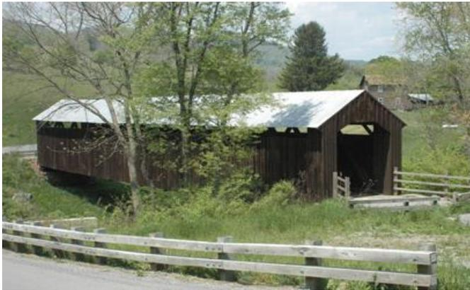
In November 2001, using special covered bridge funding provided in the TEA-21 federal highway program, a \$406,936 renovation contract was awarded to Orders Construction Company, Inc. of St. Albans that included removal of previously installed temporary supports and replacement of all materials necessary to restore it to a single-lane pedestrian structure.
