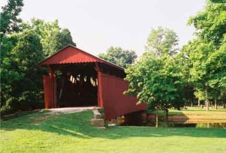
Originally crossing Tug Fork of Big Mill Creek in Jackson County, this 11.25-foot-wide, 97-foot-long Long truss bridge was built in 1888 by Henry Hartley at a cost of \$1,788.35.
