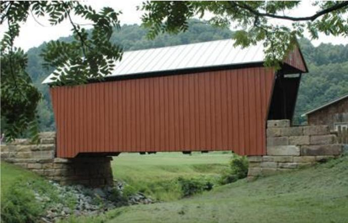
This 12.5-foot-wide, 42-foot-long Long truss built in 1889 by John Ash and S.H. Smith crosses Pike Fork of McElroy Creek just east of WV 23 in Doddridge County. No longer carrying traffic, the bridge underwent \$353,697 worth of renovations by The Righter Co., Inc. of Columbus, OH in 2002.
