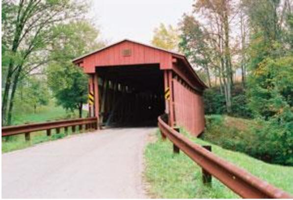
Built by R.B. Cunningham and G.W. Staats in 1890, this Long truss bridge carrying Jackson County 21/15 over Left Fork of Sandy Creek near Sandyville was dismantled and relocated 1924. The 11.75-foot-wide, 101.25-foot-long span also received some repairs in 1979.
