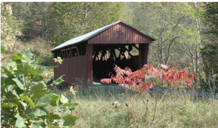
This 12-foot-wide, 81.5-foot-long Long truss, built in 1899 carries Greenbrier County 62 over Second Creek. While originally costing only \$200, renovations in 2001 by Allegheny Restoration & Bldrs, Inc. of Morgantown, WV totaled \$391,646.
